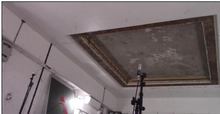
Photo No. 2 Receive Room View of Test Specimen Installation
